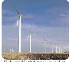
of electricity. The 3-blade, variable pitch propeller used on the Z-750 (as this latest-generation turbine is called) measures 156 ft. in diameter, and weighs 34,000 lbs! The turbines are spread over 10 square miles of farmland.
